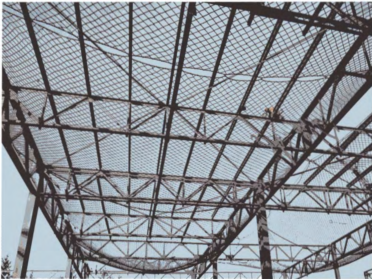
Safety Nets saved time and money on this multi-story job replacing "Boarding Over" for a fraction of the cost and with greater safety.
